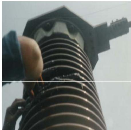
Due to flashover, the bursting of Insulators and breakage of Insulator petticoat area is a common problems in any sub station.
