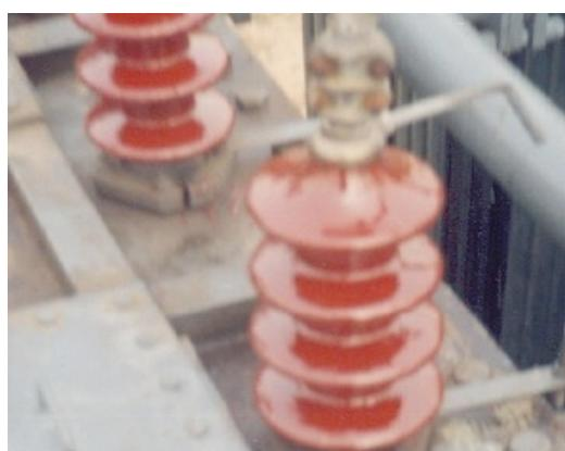
The bus bar flash over due to rat and lizards, Loss of glaze on insulator and bushings, Moisture absorption by Bus bar sprouts are the common problems faced by all the substation maintenance personnel.
